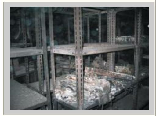
Storage room in basement of Revolutionary Command Council Headquarters. Burned frames of PC workstations visible on shelves. All rooms sharing walls with this storage
